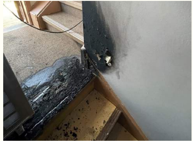
The fire damage at the top of the stairs, both the carpet and wall has been charred.
